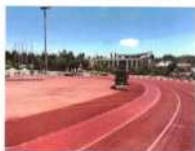
2. After high pressure cleaning immediate inspection of the synthetic surface. It is possible that high water pressure has caused the surface coating to come loose in defective or too thin areas. The entire synthetic surface should be checked after cleaning to see if there are any other areas besides the marked areas where the sports floor covering has separated from the asphalt substructure over the last 11 years. These areas should also be removed.
