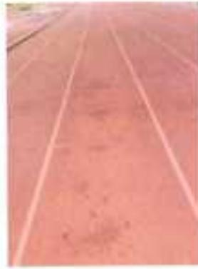
In the areas in front of the start lines for 100m, 110m and start 100m on the back straight, the upper PUR layer has expired.
